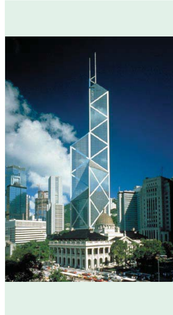
Fig. 5.4.1 The Bank of China tower in Hong Kong.
