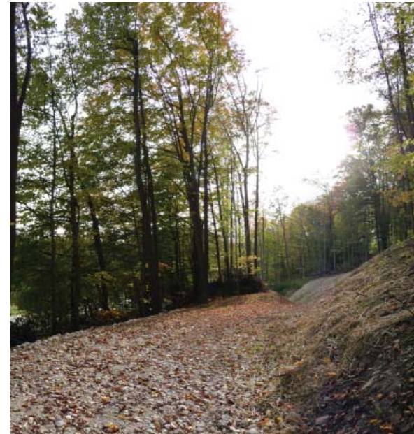
Fig. 7.7 Looking down the driving lane.
